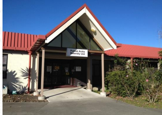
Front Entrance to Puawai Aroha Maternity Unit
